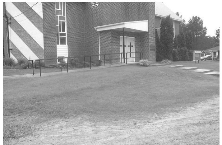
New walkway and steps
